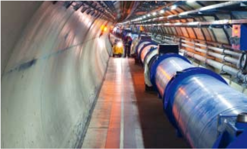
This particle accelerator is located in the 27-kilometre tunnel. Access to the tunnel is restricted and partly handled using Gunnebo entrances.
