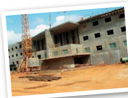
A new US embassy is being built in Riga.
