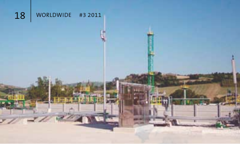
ENI has installed an integrated security solution at its new gas plant in Caparuccia.
