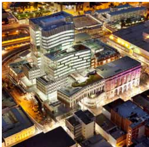
Four lanes of OptiStiles and four AutoSec doors were installed at one40william in Perth.
