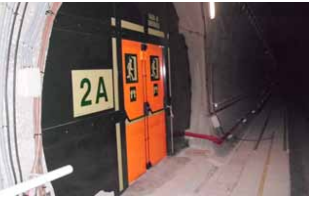
Two separate parallel tunnels, one for trains going north and the other for trains going south. In case of an emergency, passengers evacuate by crossing emergency galleries that connect one tunnel to the other horizontally every 250 metres.
