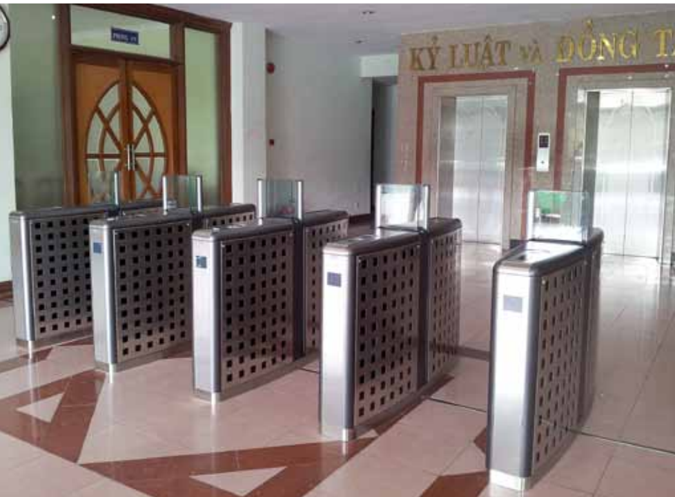
Photos: SpeedStile FP 1200 – Vinacomin Project and SpeedStile BP – VTV Project
