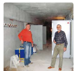
Andrzej Szymanski and Andrzej Piwonski installing vault doors in Moscow 2005.
