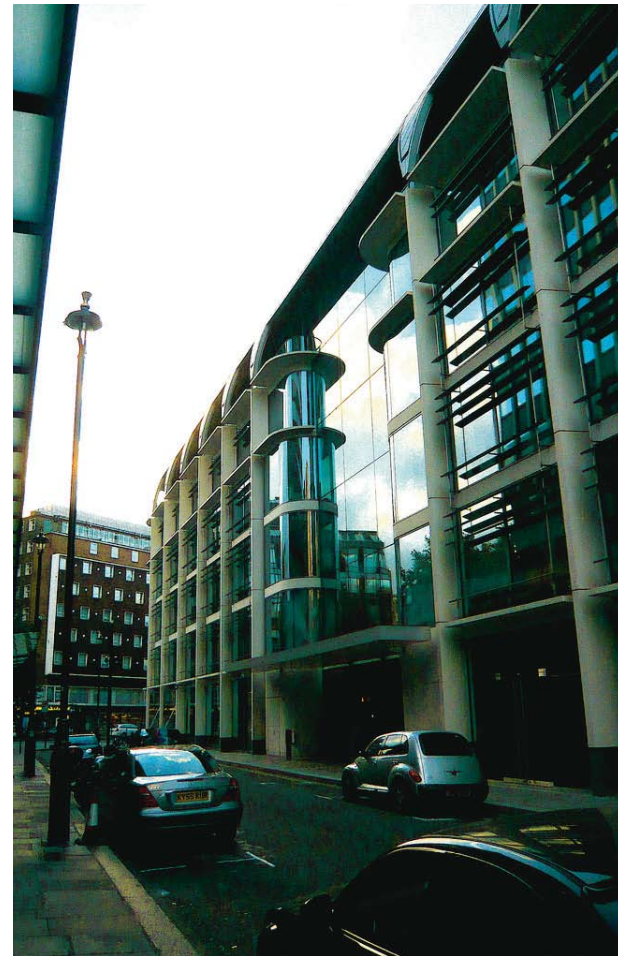
At Shaftesbury Avenue in London, Welcome Gate was brought in to review the physical safety, and it chose products from Gunnebo.
