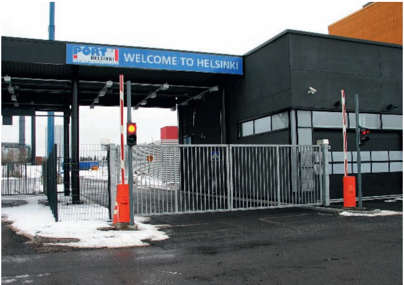
One of Finland's largest infrastructure projects in a long time is now complete: a relocation at the Port of Helsinki. Increased security requirements were one of the reasons behind the port reorganisation.
