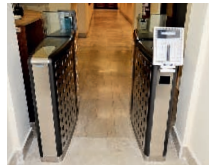
Motorised panels were chosen for access control to the Apostolic Library.
