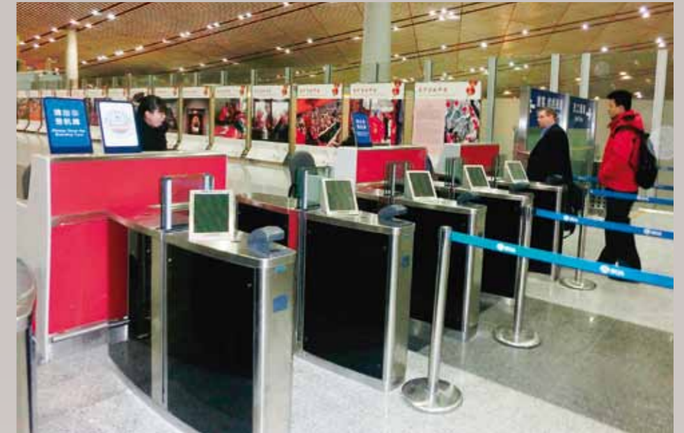
EFFECTIVE ENTRANCE. Gunnebo SpeedStile FP/FPW installed in Beijing Capital International Airport T3 can generally let through 40 passengers per minute.
