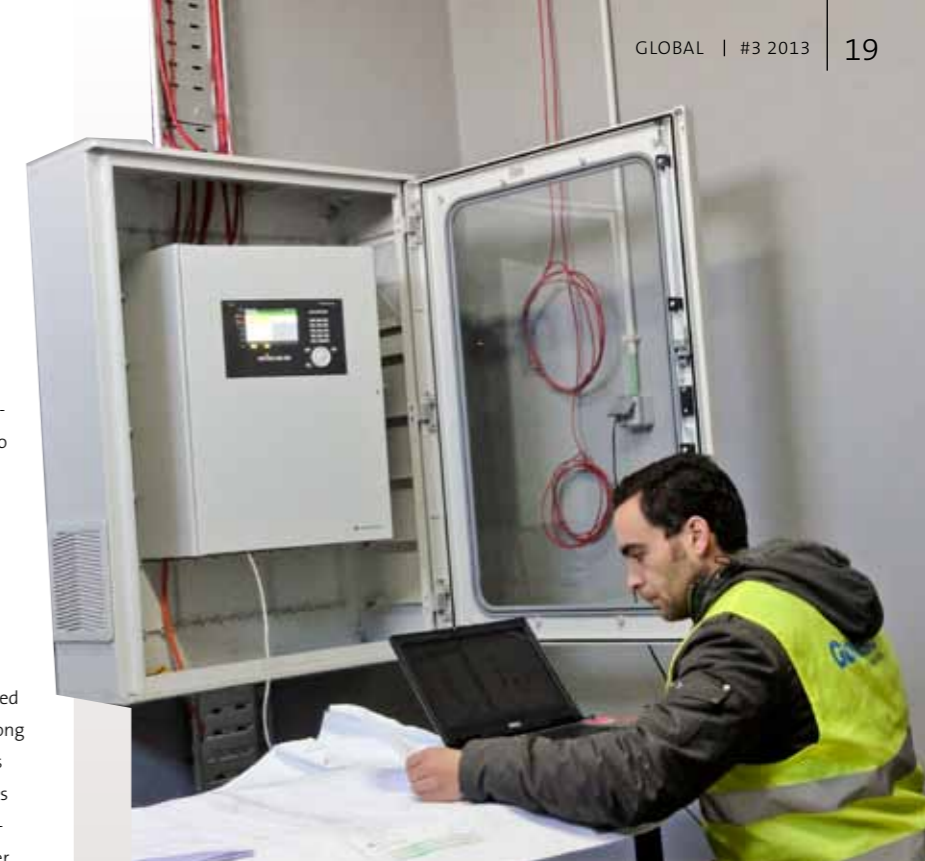
SECURITY WORK. An engineer from Gunnebo Portugal programmes the fire alarm control unit mounted on the wall.
